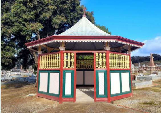
Restoration of Historic Rotundas
